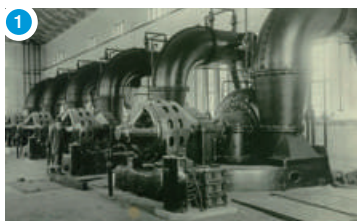
Tokyo's Asakusa Tamachi pump station
