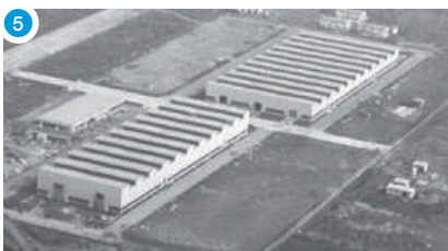
Fujisawa Plant upon completion
