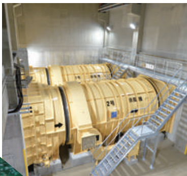
Ventilation system for the Kuriko Tunnel, Tohoku-Chuo Expressway
