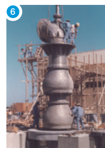
Seawater desalination pump for Saudi Arabia
